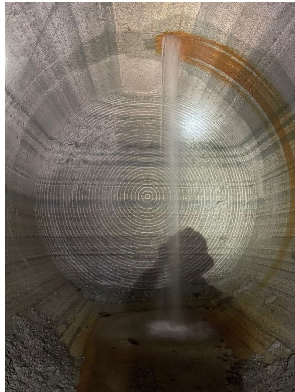
Figure 6. The end of the tunnel at Pleasant Run.
