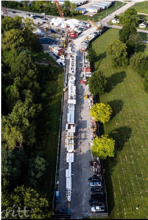
Figure 5. TBM rebuild at the Pleasant Run launch site.
