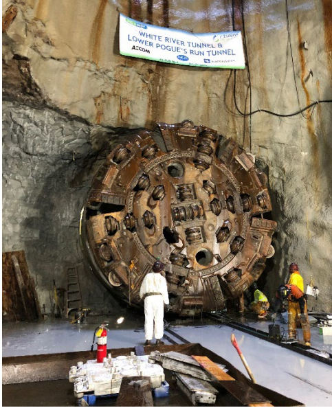
Figure 4. Breakthrough at the White River Tunnel in April 2019.
